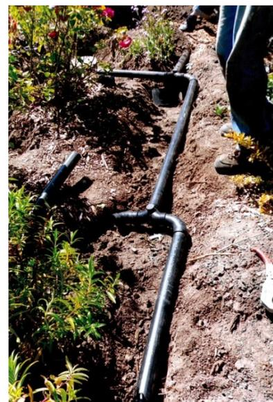
Figure 5 - Example of a ‘branched drain’ graywater system relying on gravity (source: centralcoastgreywater.org).
