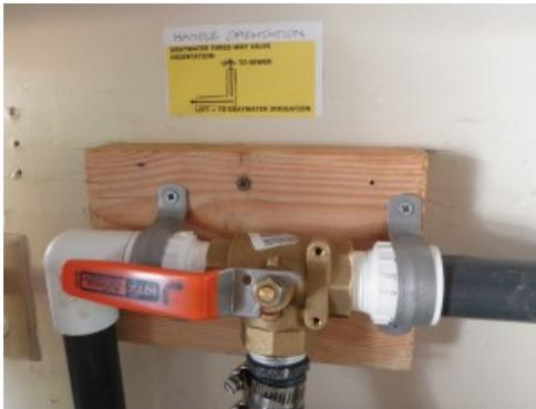
Figure 2 - A 'laundry to landscape' graywater system 3-way valve separates water destined for the sewer from water used to irrigate landscape plants (Source: <http://centralcoastgreywater.org/>)
