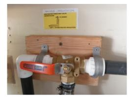
Figure 2 - A 'laundry to landscape' graywater system 3-way valve separates water destined for the sewer from water used to irrigate landscape plants (Source: http://centralcoastgreywater.org/)
