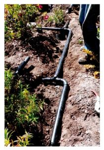
Figure 5 - Example of a 'branched drain' graywater system relying on gravity (source: centralcoastgreywater.org).
